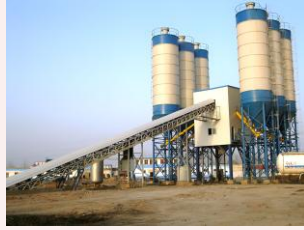
Batching Plant 1 Nos. 30 M 3
